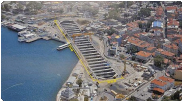
Figure 17. Marmaray Constructions in Üsküdar. ( http://i.emlak-tasovdakika.com/Files/NewsImages/900/466x255/4d9dc1ad-7bf6-42e9-a888-717169eb068a.jpg ).
