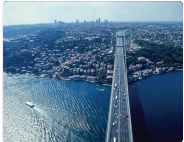
Figure 13. FSM Bridge and the European Side of İstanbul ( http://www.flickr.com/photos/58317219@N00/6838290586/lightbox/ , Photo taken by: Can Gürel).
