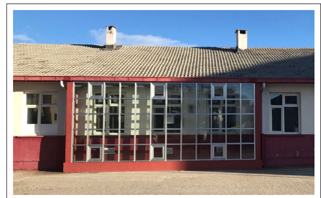
Figure 6. Applied second glass façade.
