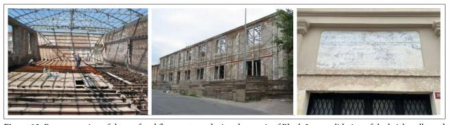
**Figure 12**. Reconstruction of the roof and floor systems during the repair of Block 2, consolidation of the brick walls, and the present state of the conserved marble inscription (Hanart Architecture Archive).
