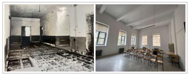
**Figure 19**. Dismantled wooden slab of the upper floor (Conservation Council Archive), Interior was reconstructed using reinforced concrete.
