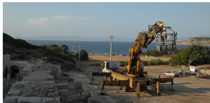
Figure 6. The use of crane to capture the site (Credit: D.G. Ozer).
