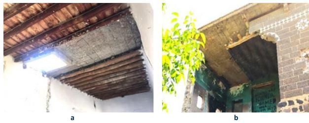
Figure 12. Deflection and material loss damages in wooden beams (Işık, 2021)
