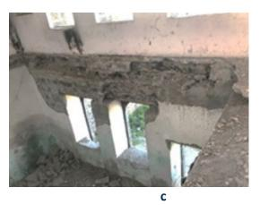
Figure 9. Ferit Köşk (Mansion) floor damages (Işık, 2021)
