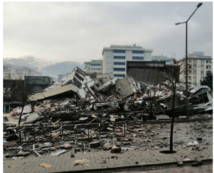
Figure 2. View of a collapsed building in the city center of Kahramanmaraş (photo by Dr. Yavuz Orak).
